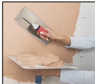
PLASTER over Plaster-Grip Primer.
